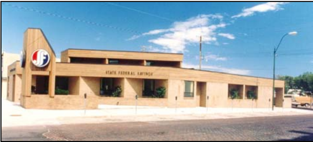
State Federal Savings - York, NE
